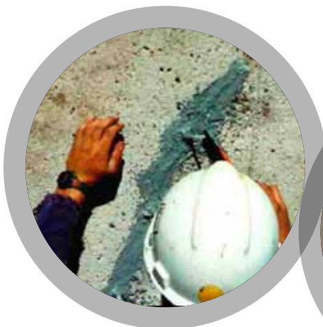
Crack Stabilization
