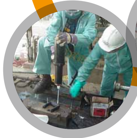
Base Plate Grouting
