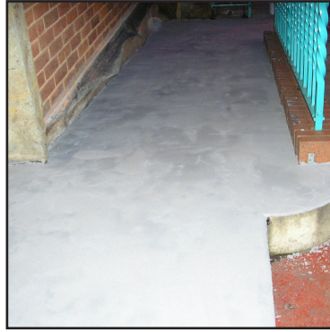
Surface rebuilt with Belzona® 4131
